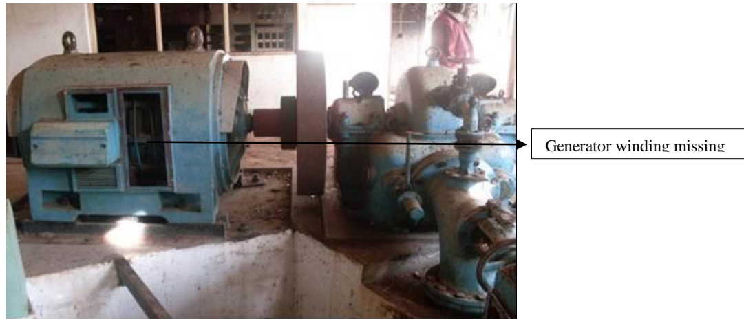
Figure 2.3 Damaged synchronous generator
