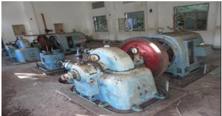
Figure 2.2 Damaged turbines and Generators
