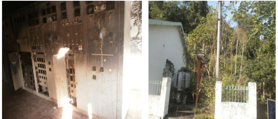
Figure 2.4 Burnt electrical switch board and damaged transformer
