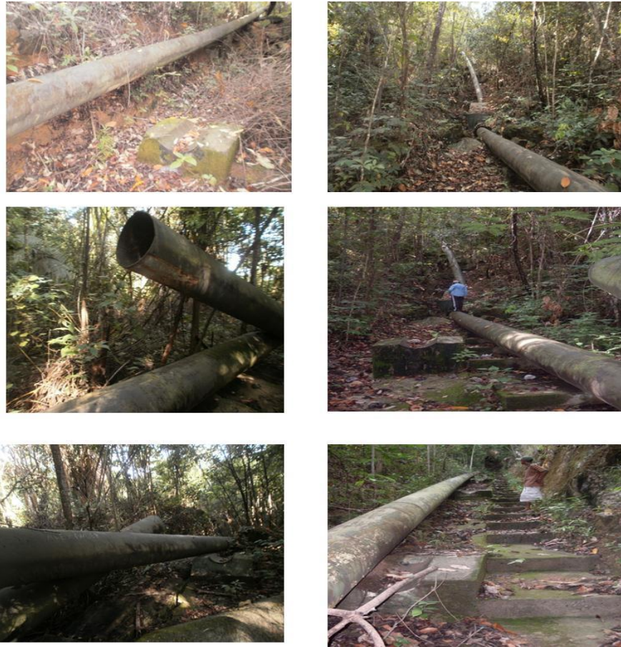
Figure 2.1 Images of Damaged penstocks
